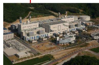
2013 Dongdoocheon CCPP (1880 MW) KOR, 185 m 3
