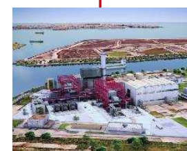
2023 Maghera Levante powerstation Veneto/IT, 57 m 3
