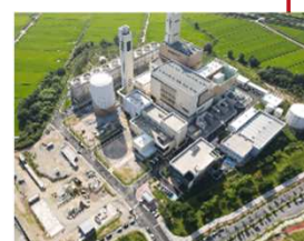
2022 Naepo District Heating Plant (500 MWe) Naepo City/KOR, 63 m 3
